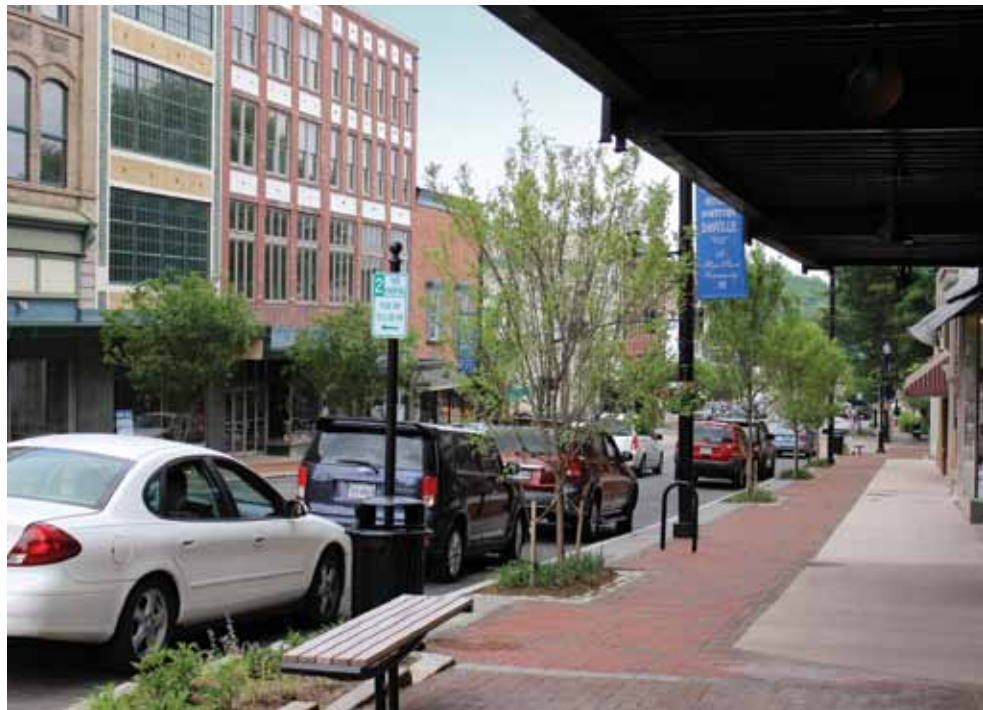
Along a portion of Main Street the city widened sidewalks, installed brick pavers, created safer pedestrian crossings, upgraded utilities and placed trees, benches and new lighting.
