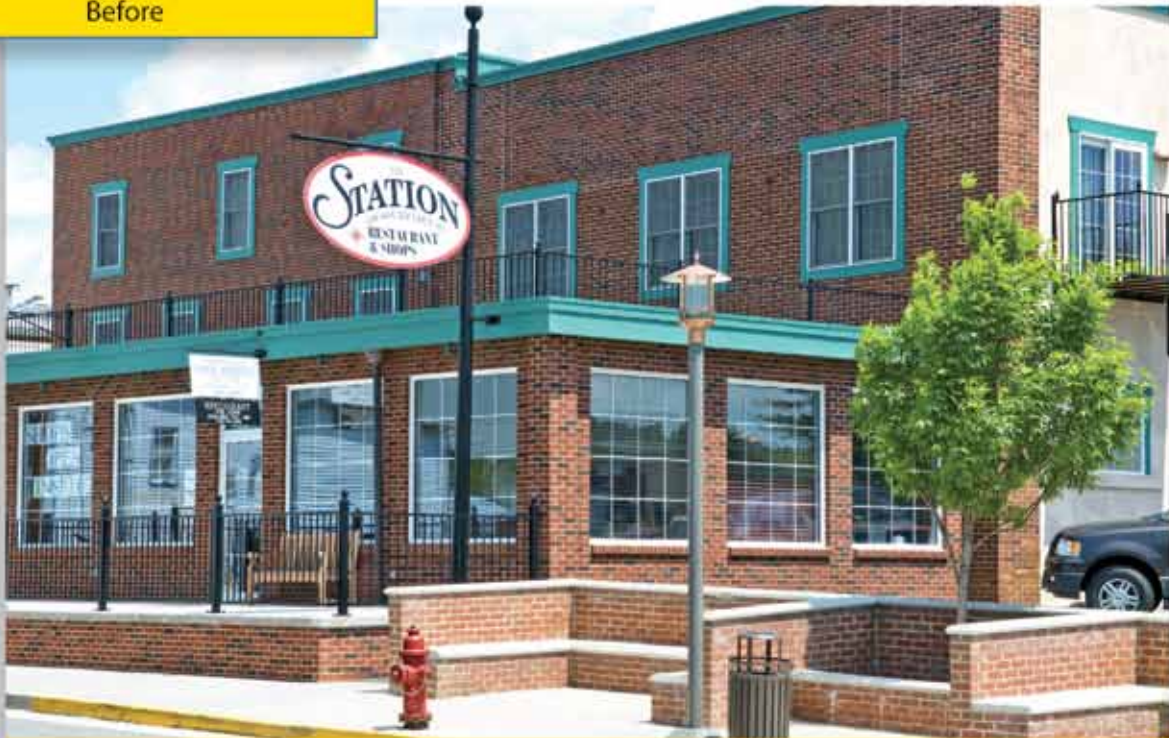
After - The Station on South Locust, Floyd, Virginia
