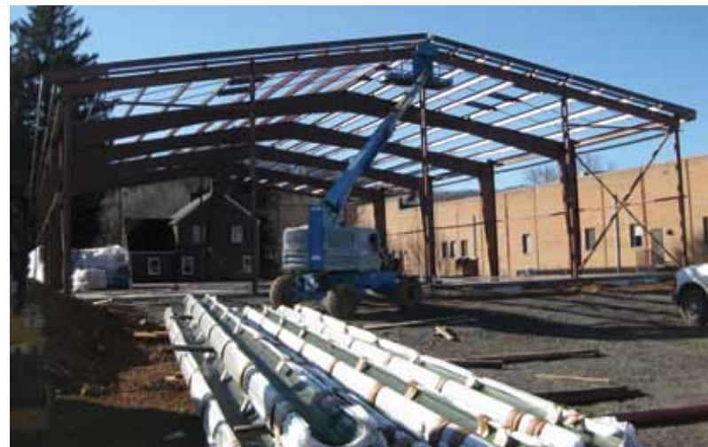
The depot was rebuilt to exacting historical standards.
